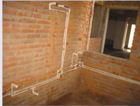
Internal Brick partition & plumbing work of Tower1(WESTAR RESIDENCY, BALKUMARI)
